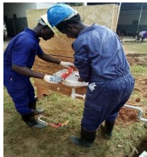
PLUMBERS (STUDENTS) INSTALLING A HAND WASHING BASIN AS PART OF THEIR PRACTICAL EXAMINATIONS DURING DIT ASSESSEMENT.
