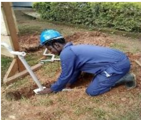
PLUMBING STUDENT FIXING A NIPPLE FOR WASTE -WATER FOR HAND BASIN DURING DIT EXAMS
